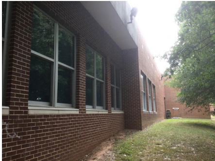
7). Northwest Elevation - Dec 16, 2019
