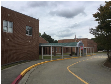
4). East Elevation - Dec 16, 2019
