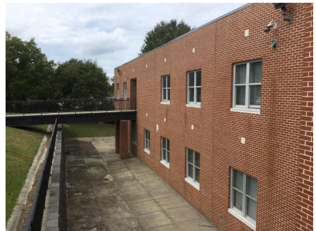
9). Southwest Elevation - Dec 16, 2019
