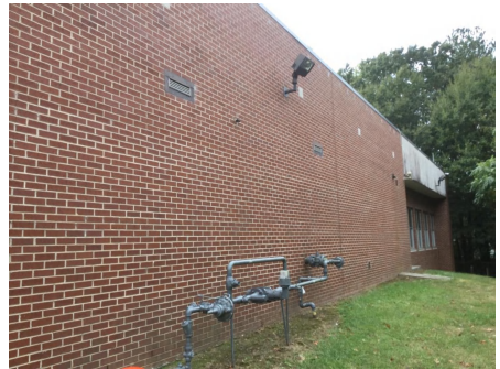
6). North Elevation - Dec 16, 2019
