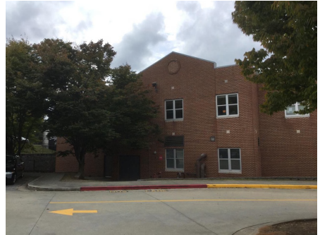
3). East Elevation - Dec 16, 2019
