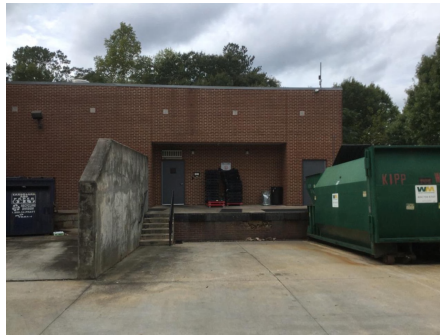
5). Northeast Elevation - Dec 16, 2019
